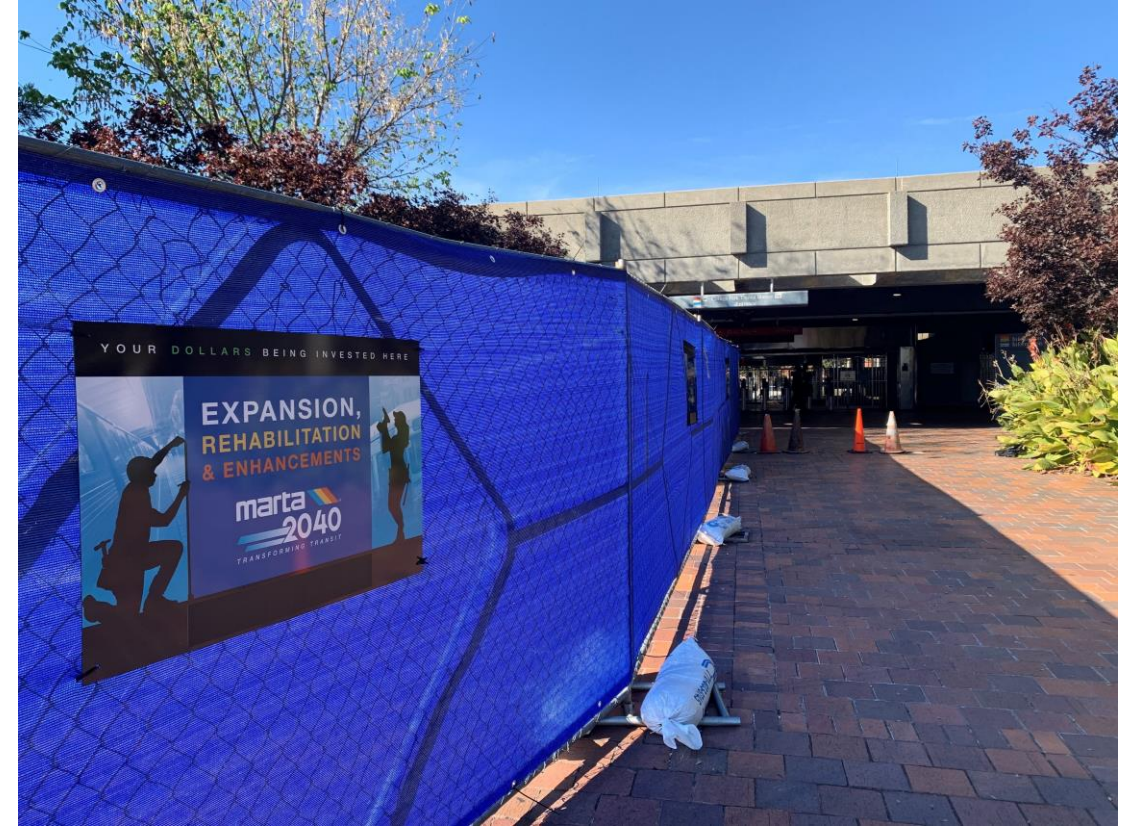
College Park Station Rehab – Expected complete 2022
